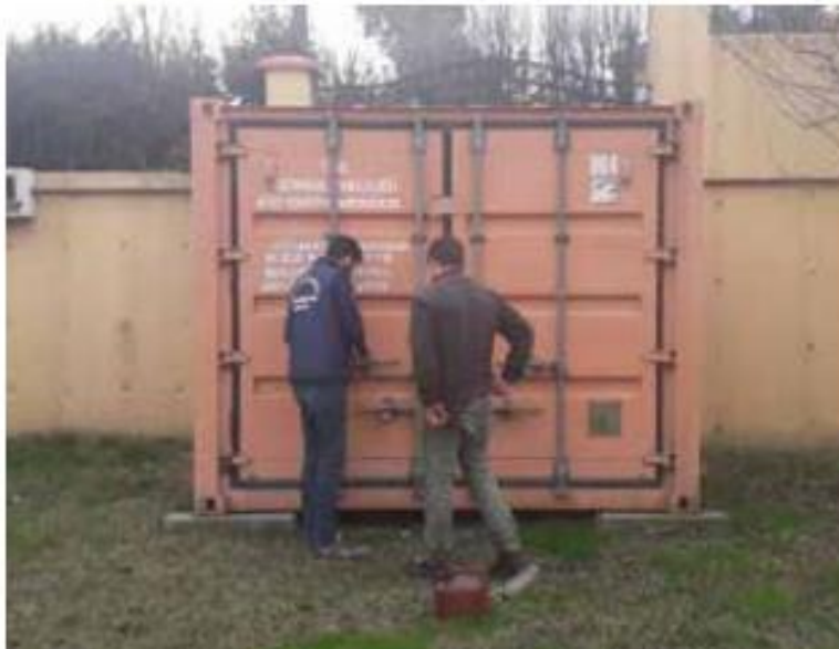
Figure 8. AFİS Container Works
