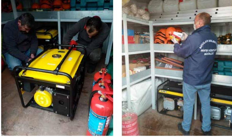
Figure 9. AFİS Container Works-1
