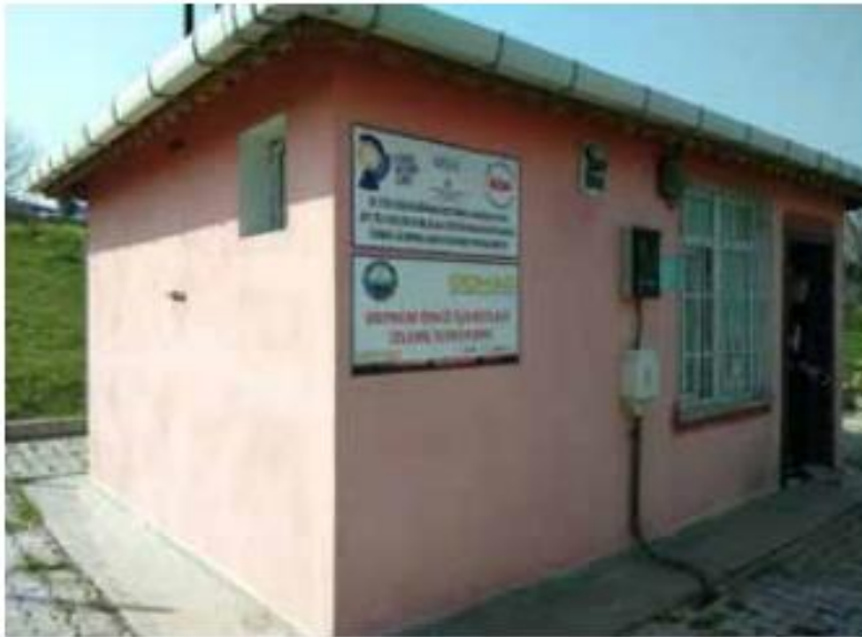
Figure 6. Earthquake Precursors Observation Station
